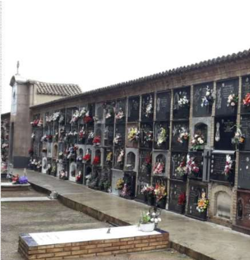
6. Vista general del interior
